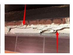
GAS LINE 10: Gas Line: Potential Hazard Gap Around Gas Line
